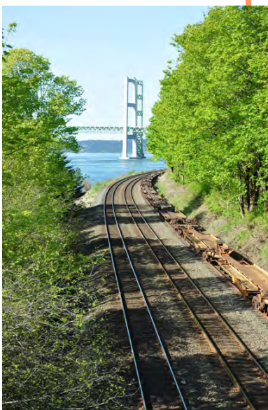
Rail near Titlow Park
