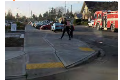
Recently completed sidewalk at Safeway site in Proctor
